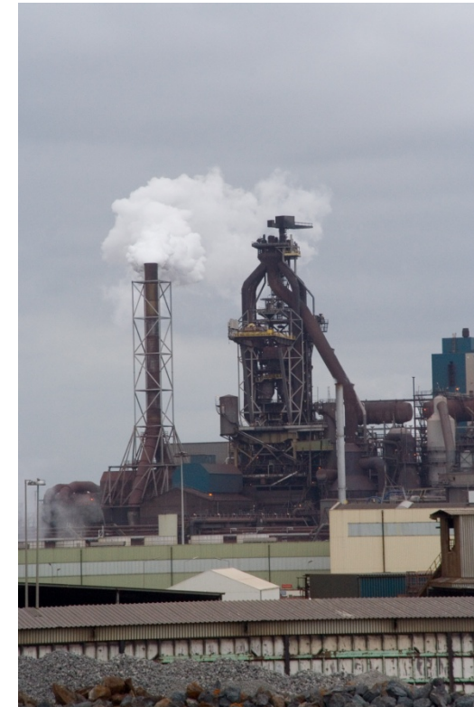
Figure 1. A blast furnace at Ijmuiden, in The Netherlands. It uses coke to reduce iron ore into iron. The parent company is part of ULCOS, a group investigating how to capture the emissions from the blast furnace and how the entire process might be electrified through the use of electrolysis rather than chemical reduction. Photo © Svdolen.
